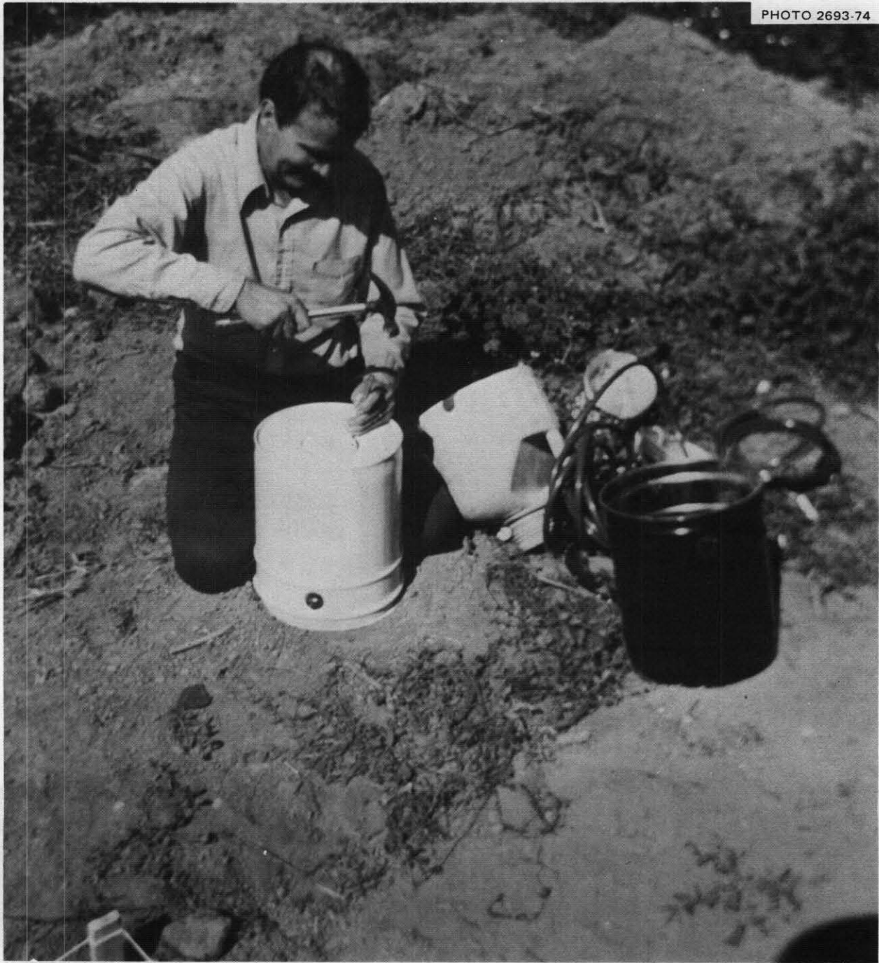
Fig. 4.25. The father starting work, with cold chisel and hammer, on his clever design of an odorless expedient toilet. In order to determine how long it would take to build and install this toilet under field conditions, he brought from his home the two 5-gallon cans, a 5-gallon plastic water jug (shown upside down), a garden hose, a complete toilet seat, an uncut piece of plywood, a tube, some cord, and freezer tape – all the materials needed to build this toilet.
